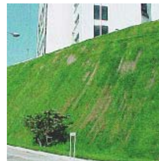
Adjacent Slope of the hospital : Monotonous shotcreted slope treated with toyo mulching to achieve greening effect.
