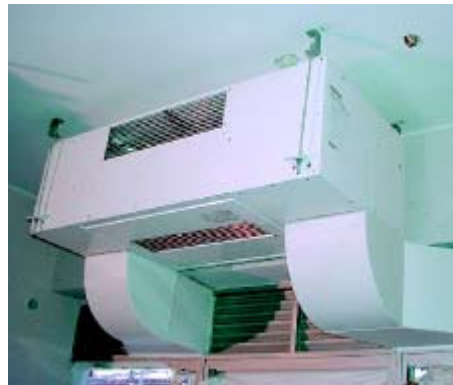
Fresh Air Pre-conditioner installed above corridor of school (Left) and the appearance of the equipment (Right).
