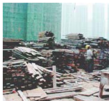
Timber formwork piled up for re-use on site.
