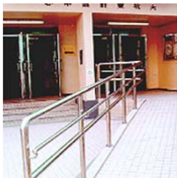
Access ramp to building entrance.
