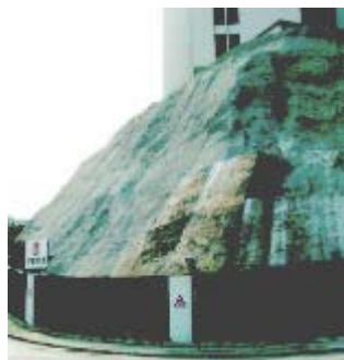
Adjacent Slope of the hospital : Monotonous shotcreted slope treated with toyo mulching to achieve greening effect.
