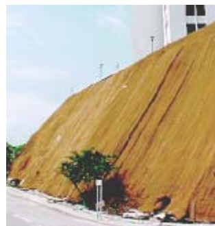
Adjacent Slope of the hospital : Monotonous shotcreted slope treated with toyo mulching to achieve greening effect.
