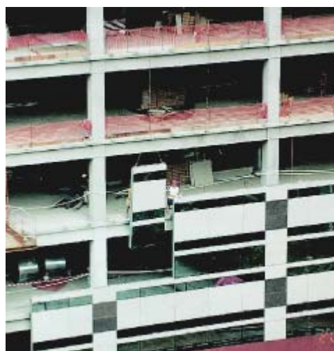
Installation of the unitized curtain wall system on site.
