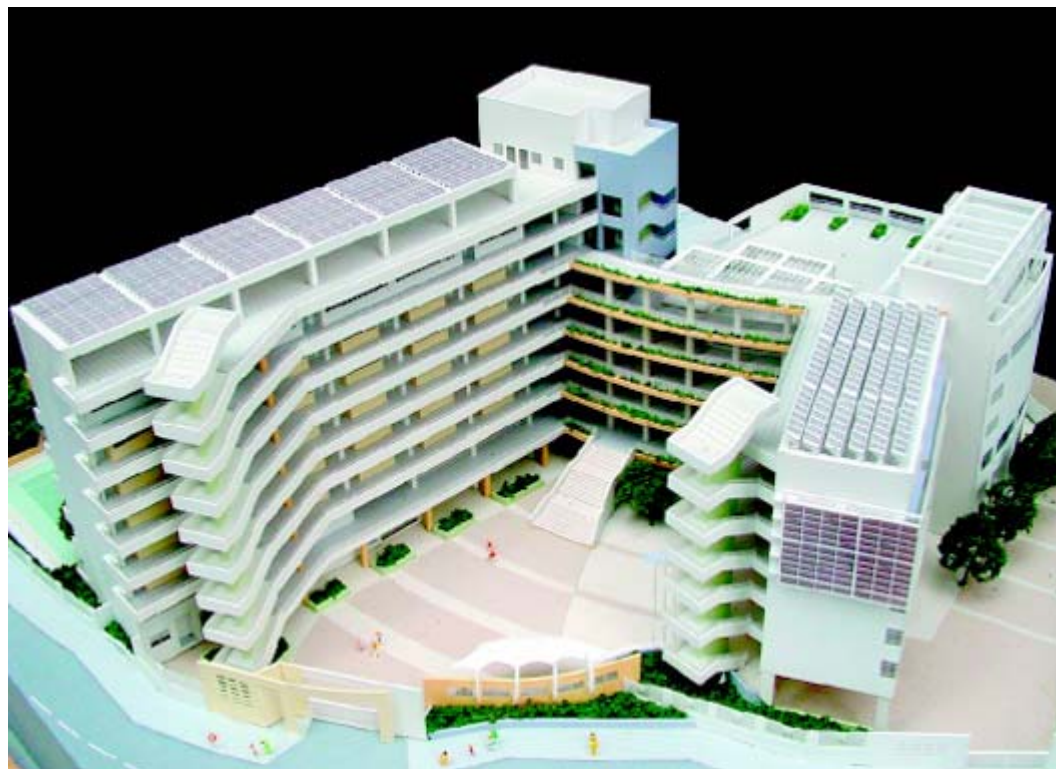
Proposed BIPV Panels to be installed on the roof and the western elevation of Ma Wan Primary School
