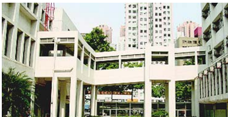
Addition of footbridge and lift tower at a new school block to link up to the rest of the existing school compound.
