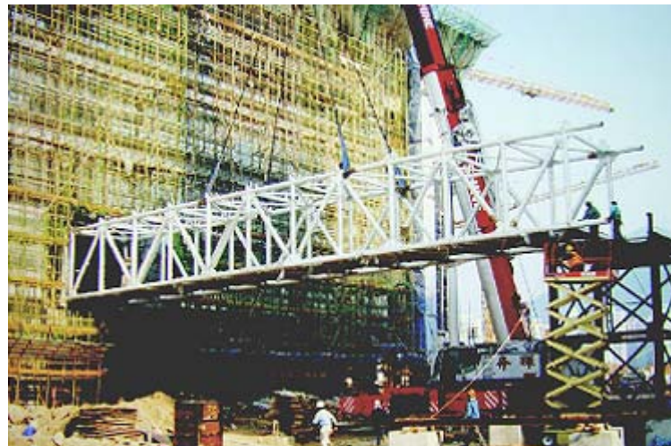
Science Park Footbridge Construction
