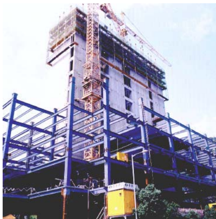
Hybrid structure under construction.
