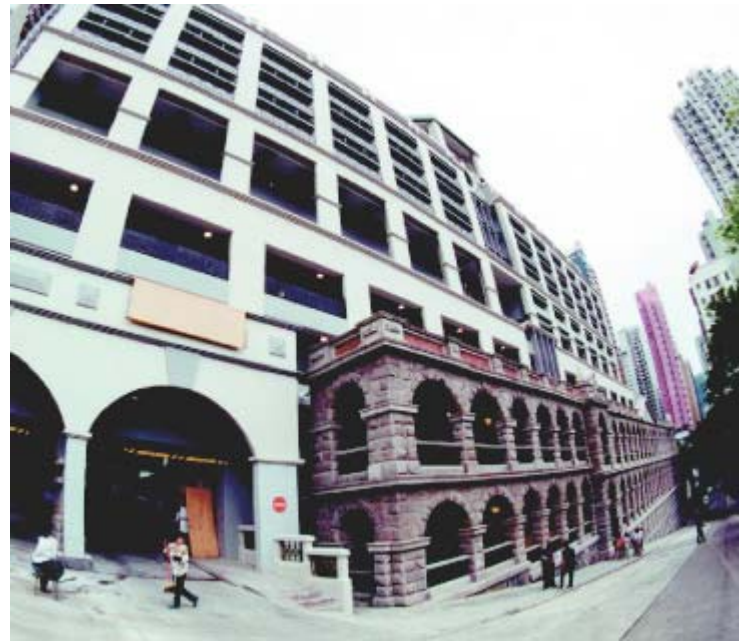
A new community centre and a singleton hostel was constructed behind the old façade with historical heritage.
