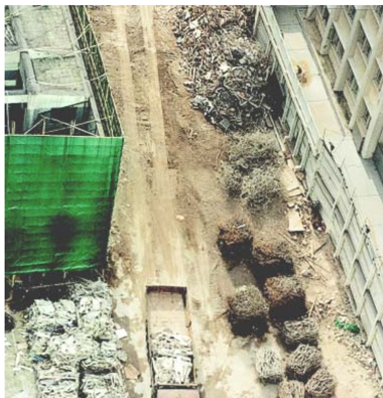
Demolition of Police Headquarters – Implementation of waste sorting on site.
