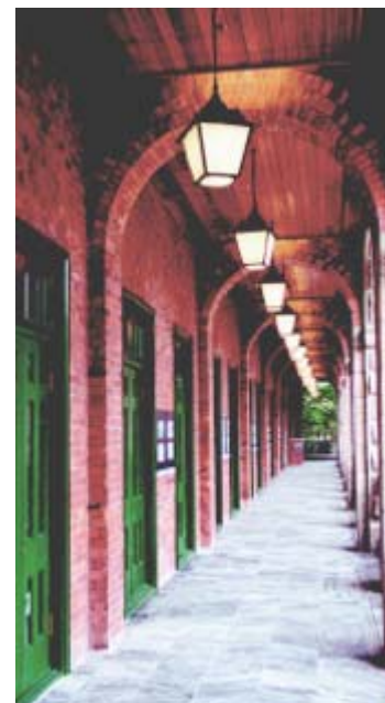
The verandah after restoration.
