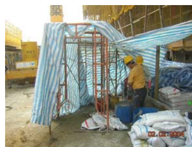
Shelter was provided during dusty operation
