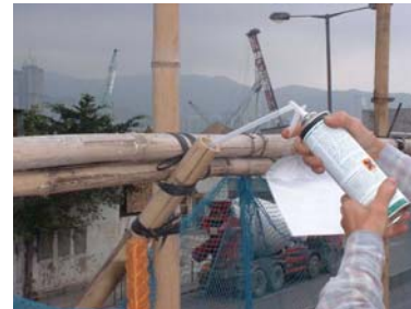
Expansion foam was applied to bamboo nodes to prevent accumulation of stagnant water
