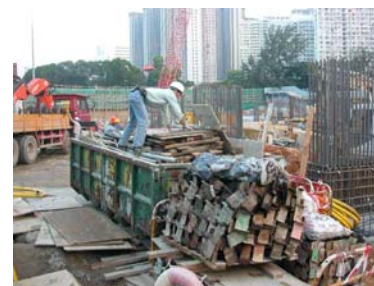
Systematic sorting for re-use or recycling of construction materials
