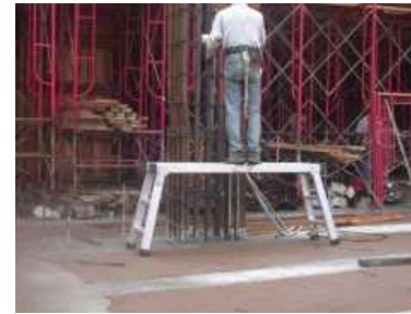
A safe working stool for fabricating steel cage
