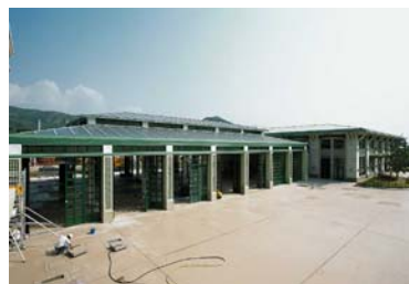
Fire Station before handover (Gold Award).
