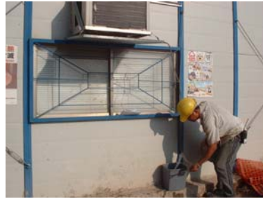
Clearing site office drainage system - an anti-mosquito measure
