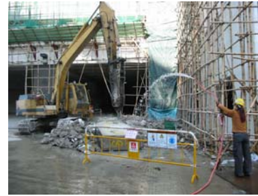
Dust control with water during breaking of demolished concrete panel
