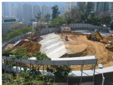
A site with excavation commenced
