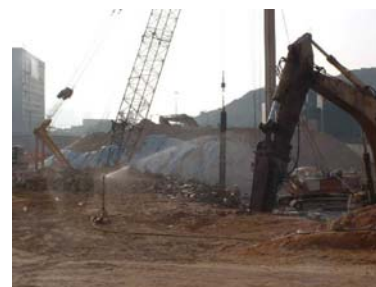
Dust control during rock breaking using water sprinklers
