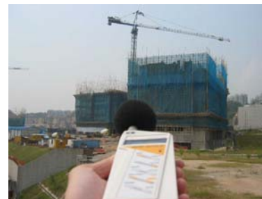
Regular noise assessment at a school neighbouring construction site
