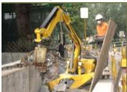
Reducing noise pollution by the use of pneumatic concrete breaker
