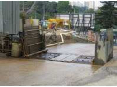
Water recycling facilities and automatic wheel washing system at site entrance
