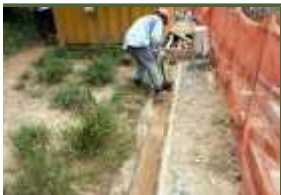
Removal of blockage at surface channel on site
