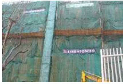
Fully enclosing the material hoist for dust suppression
