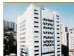
Urban Council Sheung Wan Complex (1989)
