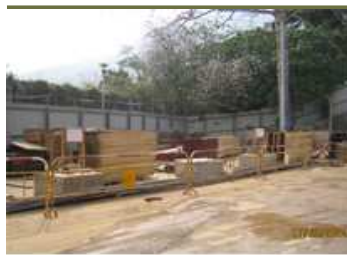
Timber formwork and lumbers were sorted for future re-use
