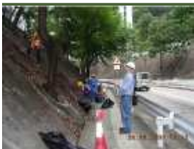
Slope inspection by ArchSD staff
