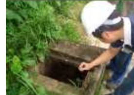
Inspection of manholes by ArchSD staff
