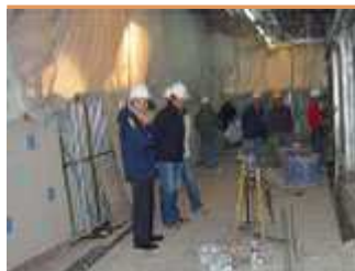
Site Safety Inspection
