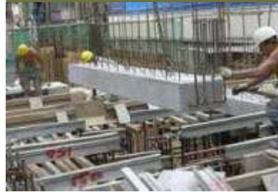
Extensive use of precast concrete elements in the superstructure
