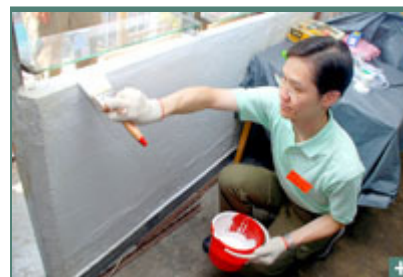
We repaired the home of some elderly
