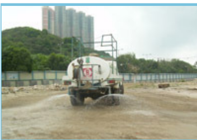
Dust control measures on site
