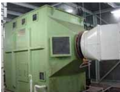
Water scrubber system to reduce odour nuisance
