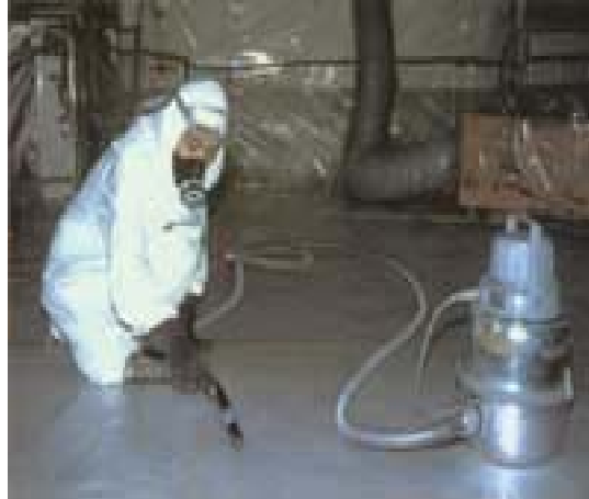
Vacuum cleaning asbestos materials
