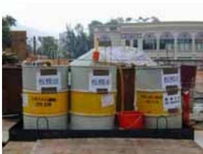
Proper containment of hazardous materials to avoid contamination
