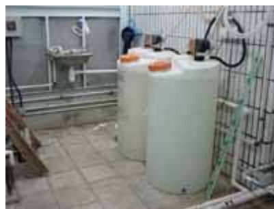
Water scrubber system to reduce odour nuisance
