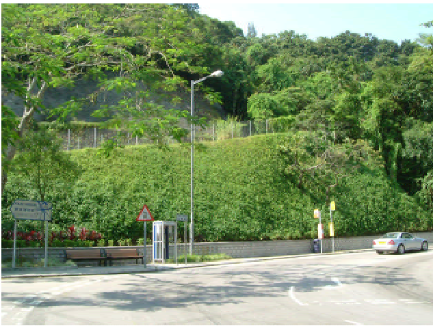
An example of the use of a Group 1 technique/product - Geofibre
