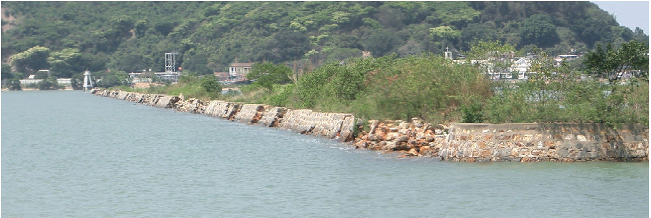
General condition of the historic seawall
