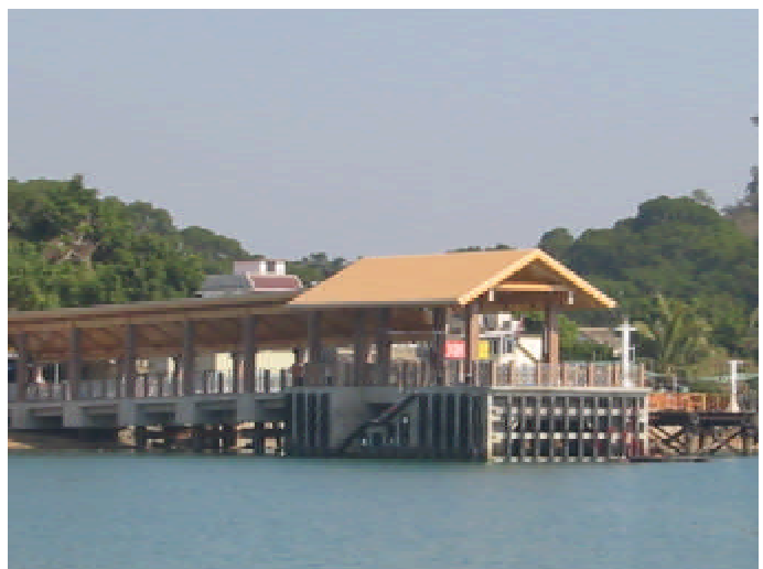
Timber pitched roof cover system at Kat O Chau Public Pier
