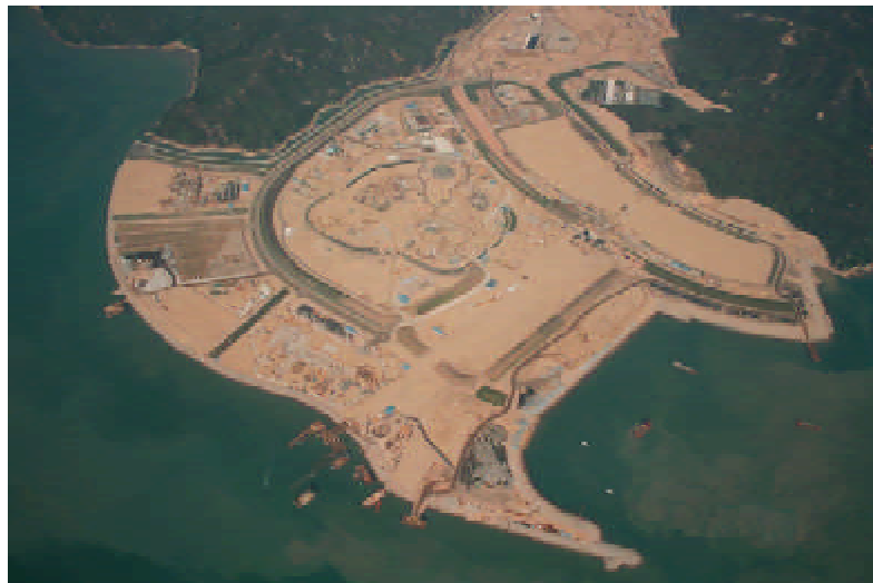
General view of Penny's Bay Reclamation site
