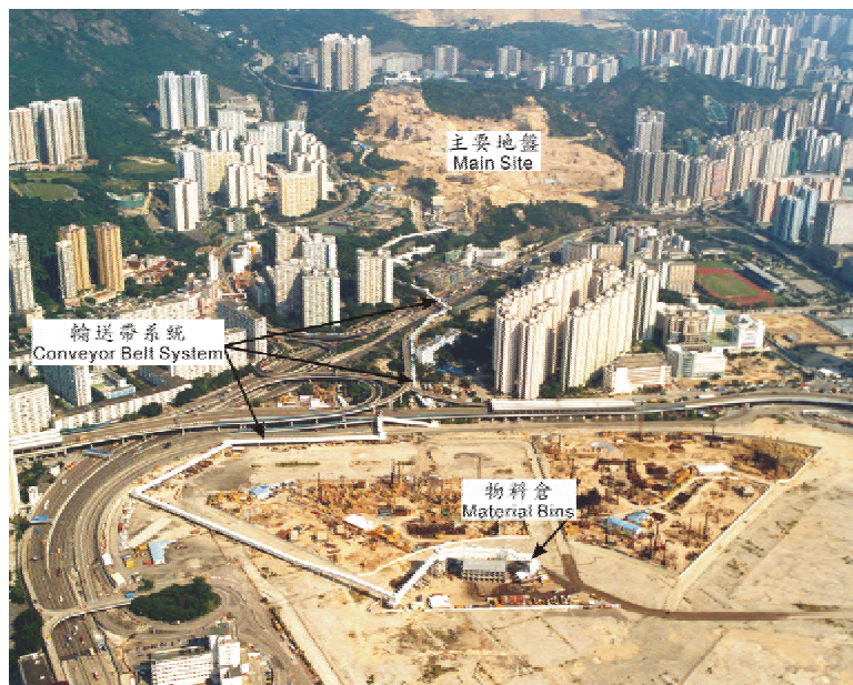
Site formation at Choi Wan Road and Jordan Valley - Conveyor Belt System
