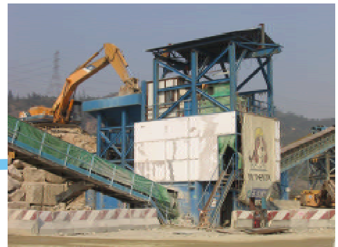
Crushing and Sorting Yard
