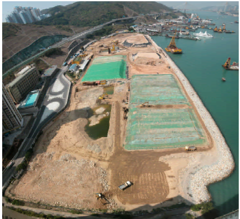
The biopile (shown green) soil treatment at North Tsing Yi
