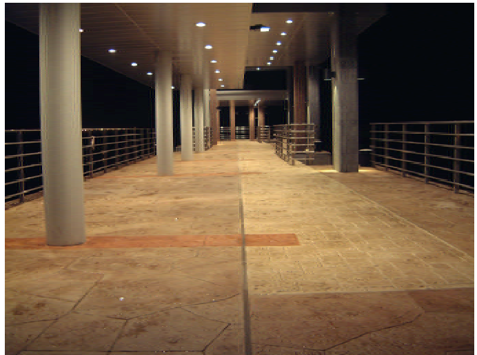
Application of imprinted colour concrete with different granite patterns at Peng Chau Public Pier
