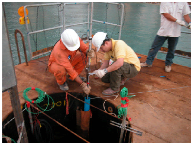
Installation of the geotechnical monitoring instrumentation
