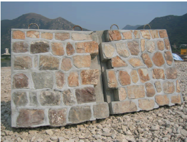
Trial facing panel of seawall using existing facing stones
