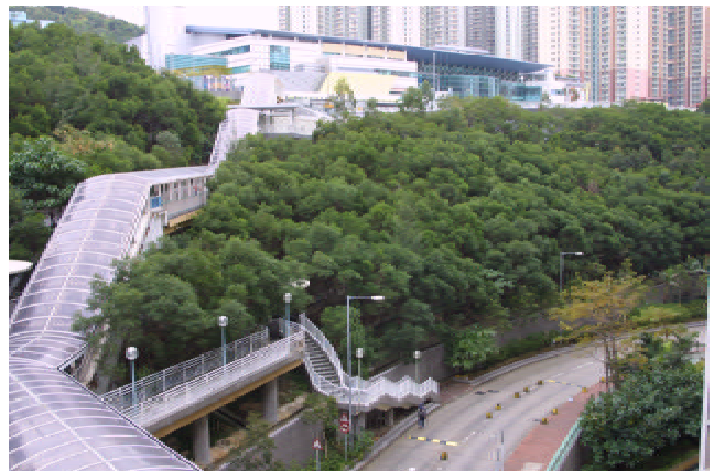
1st runner-up slope at Sau Mau Ping Estate III
