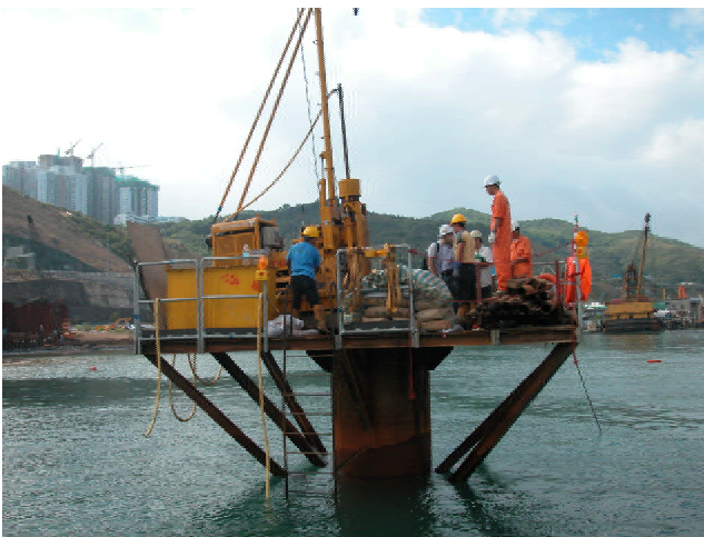
Arrangement of working platform for geotechnical monitoring instrumentation
