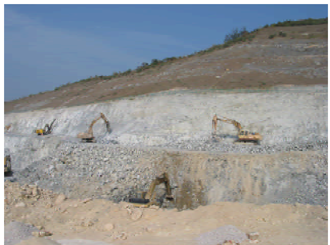
Rehabilitation of Anderson Road quarry
