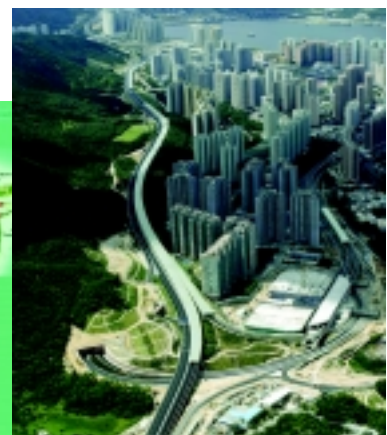
從北面俯瞰 T7 號道路 Aerial View from North
