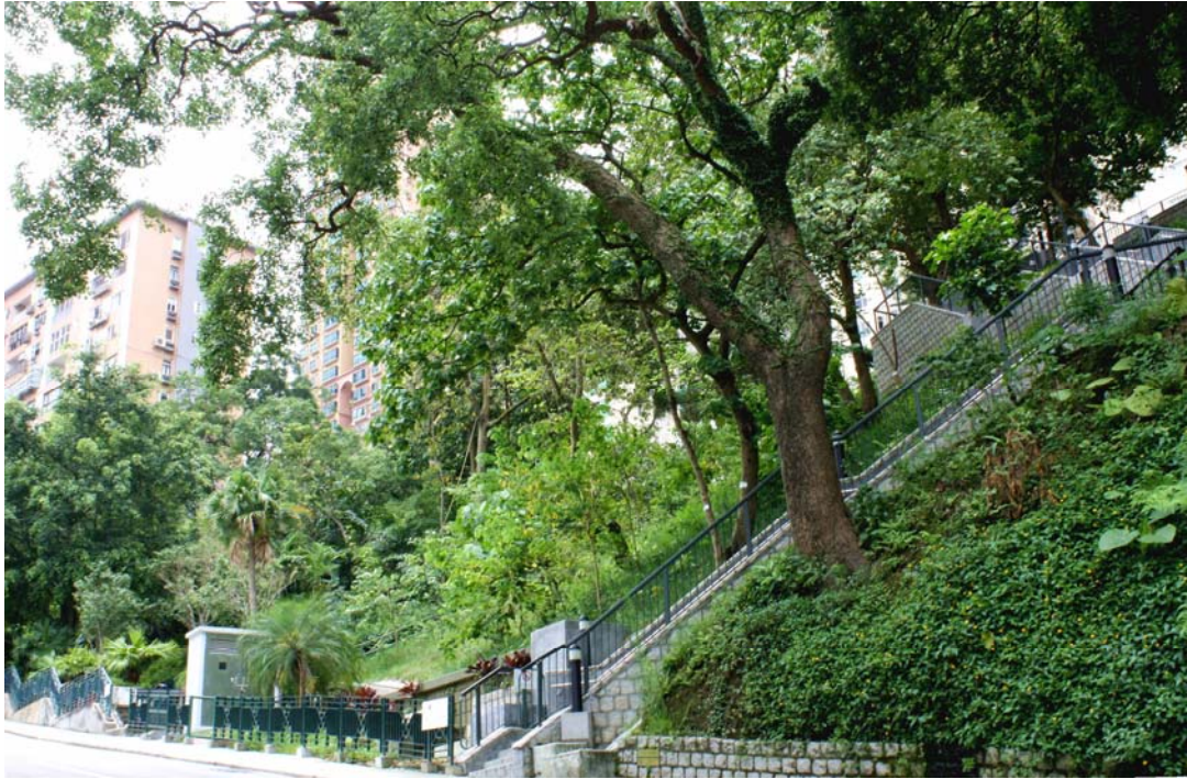
A man-made slope upgraded and greened under the LPM Programme
