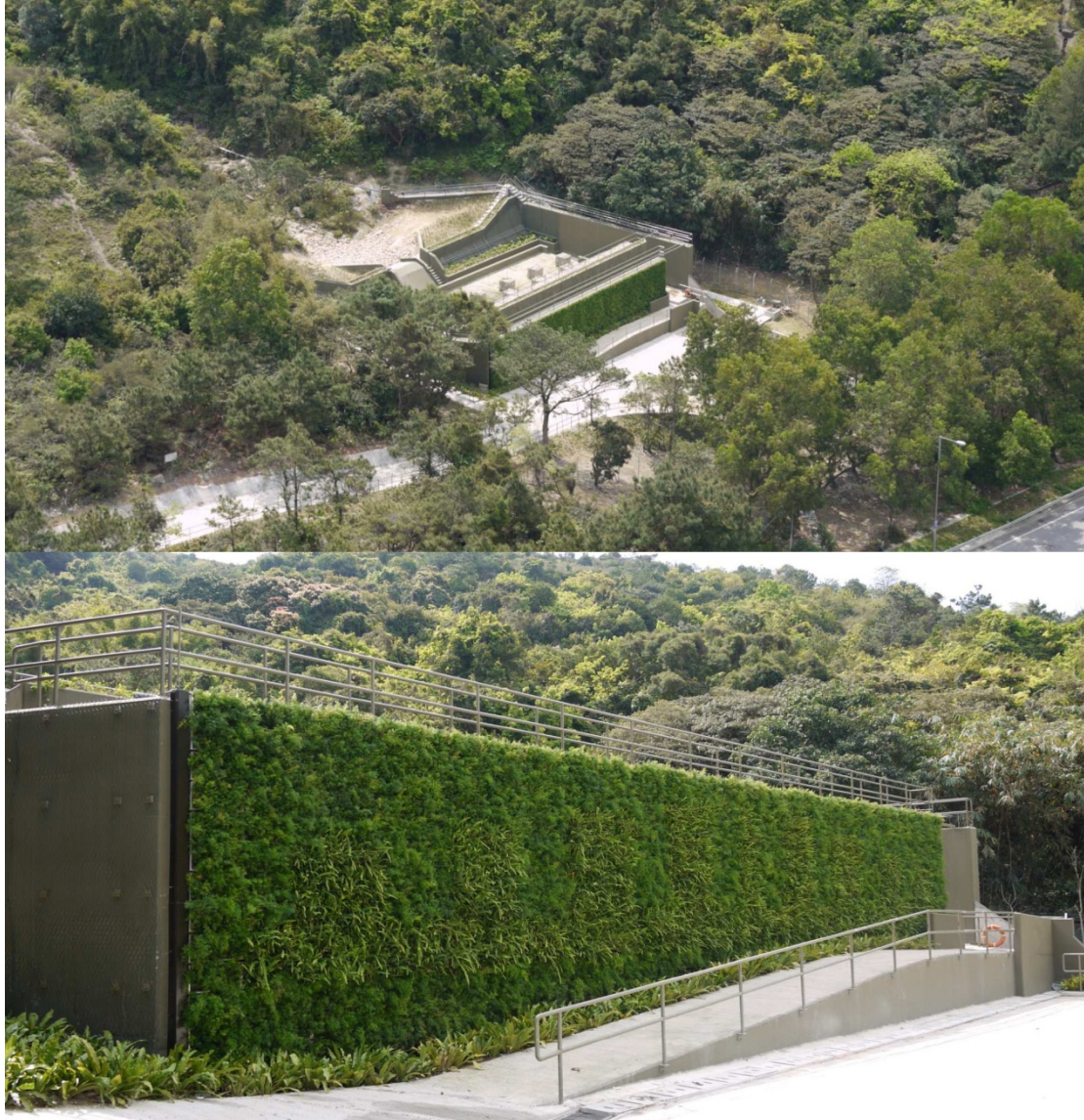
Landscape treatment of natural terrain under the LPMit Programme
