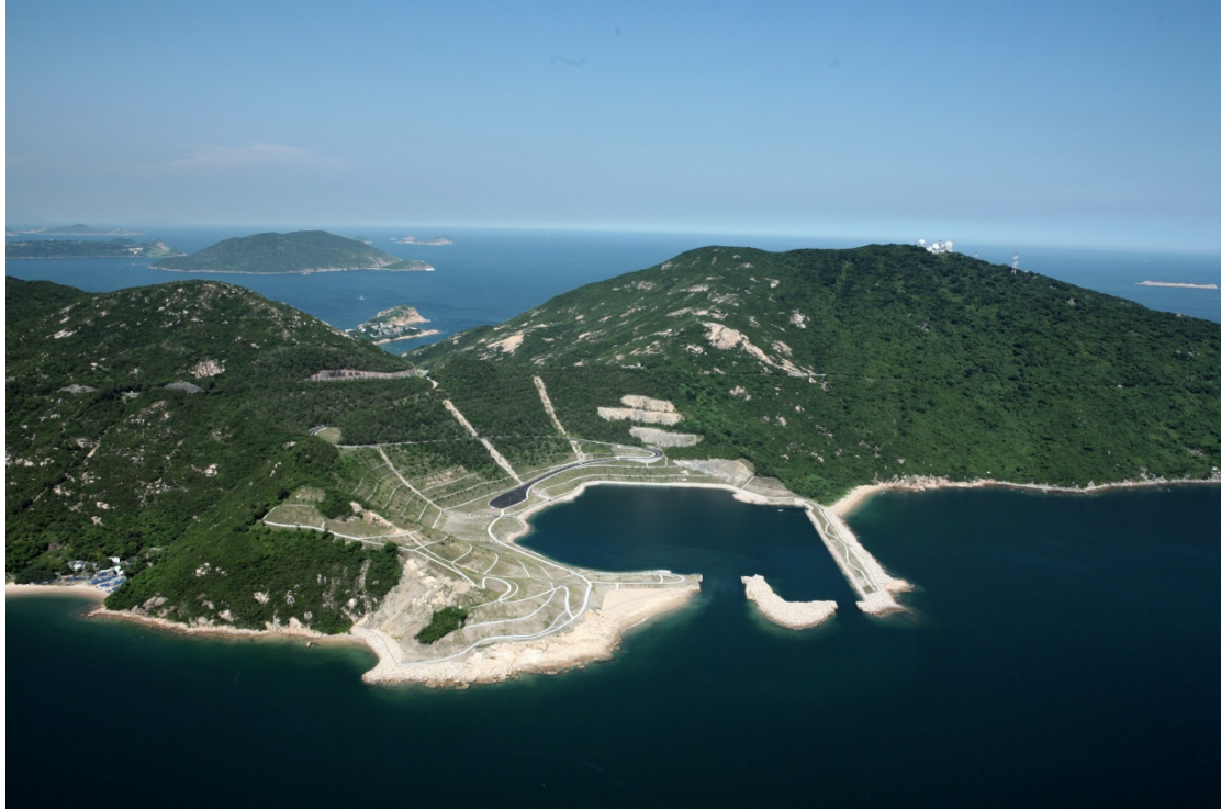
Aerial view of rehabilitated Shek O Quarry
