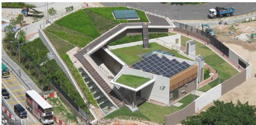
Green roof at Kowloon City Pumping Station No. 1.
