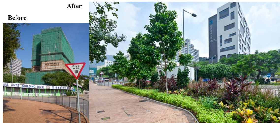
Greening works under the GMP for Wong Tai Sin - Yuk Wah Street
