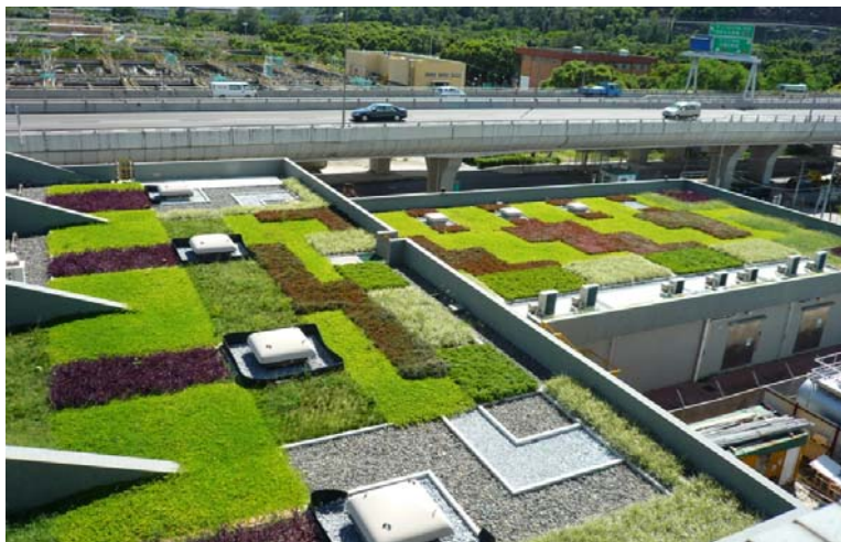
Roof greening at Shatin Sewage Treatment Works
