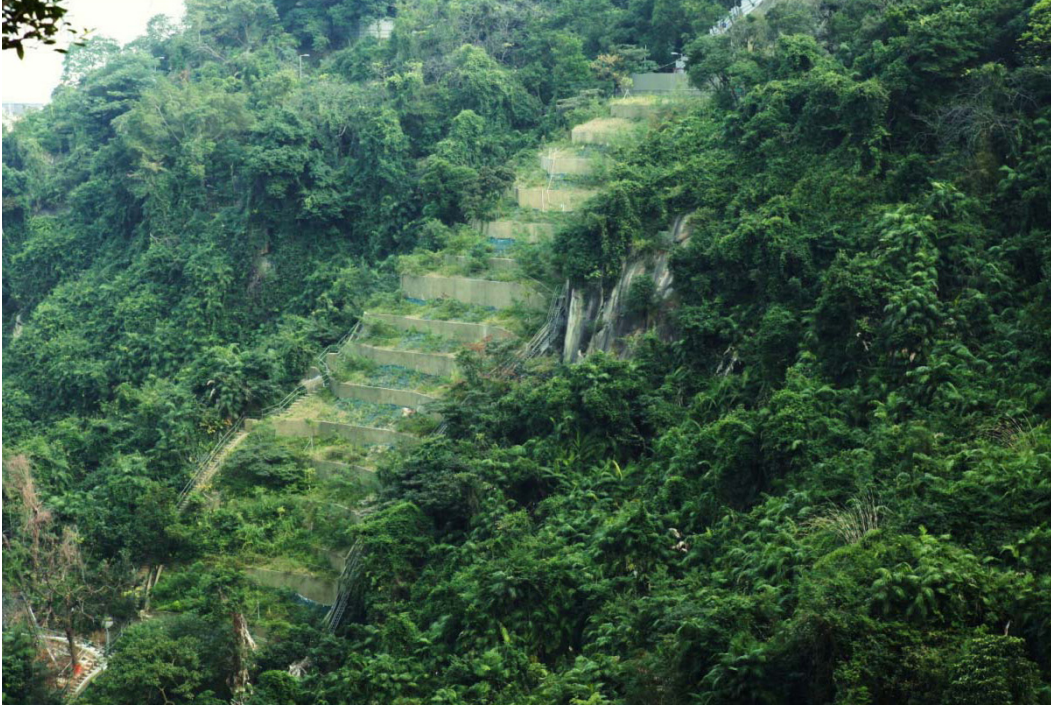
A landslide scar stabilised and greened under the LPM Programme
