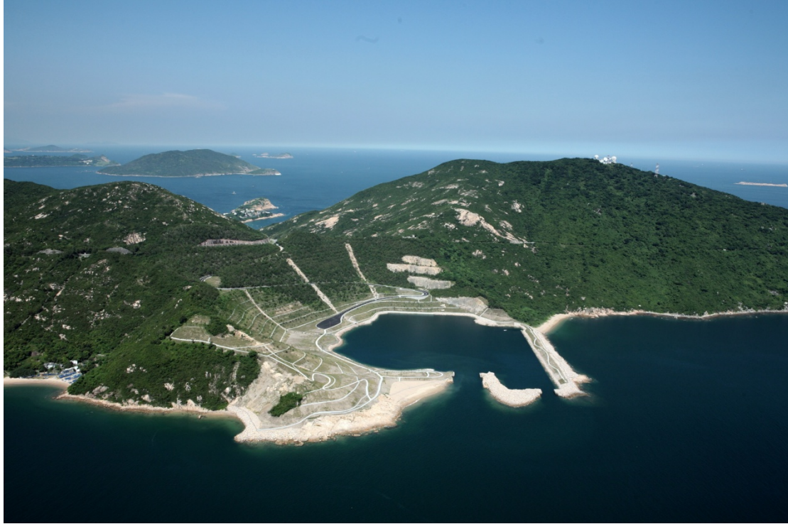
Aerial view of rehabilitated Shek O Quarry
