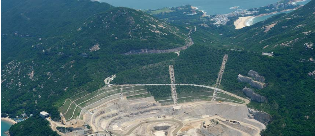
Shek O Quarry rehabilitation work in progress
