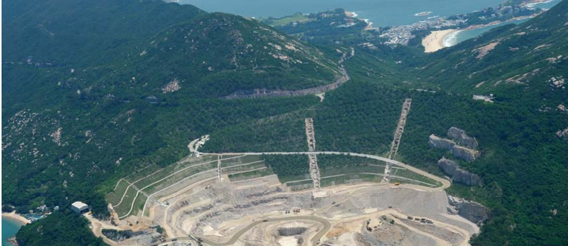
Shek O Quarry rehabilitation work in progress
