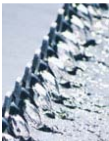
Purified effluent from final sedimentation tank
