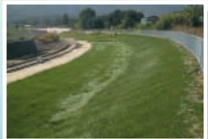
植草後的一段梧桐河河堤和河床 Grassed embankment and channel bed at River Indus
