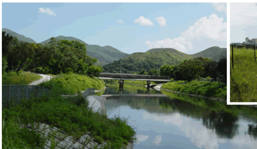
Grass-lined side slope at River Beas promoting the regeneration of riparian habitat.
