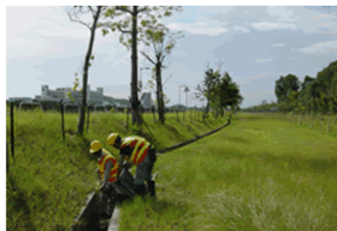
Grassed levee along Shan Pui River
