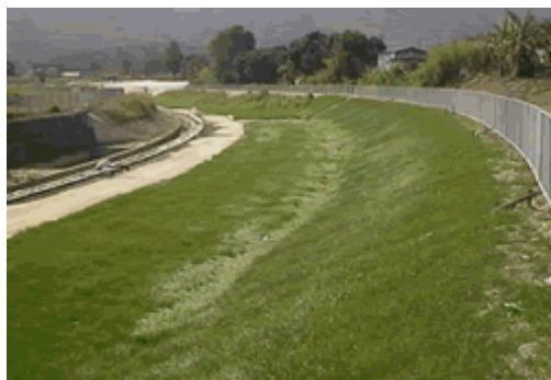
Grassed embankment and channel bed at River Indus
