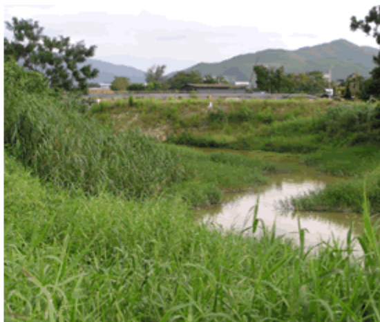
Grassed levee along Shan Pui River
