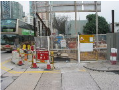
Works in Java Road near North Point Pier
