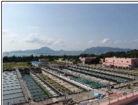
Siu Ho Wan Sewage Treatment Works
