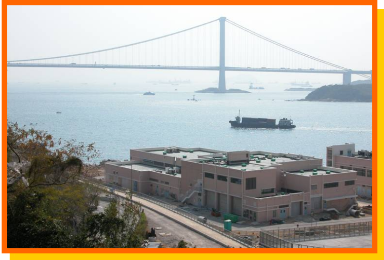
Chemically enhanced primary treatment has been implemented at the Sham Tseng Sewage Treatment Works.
