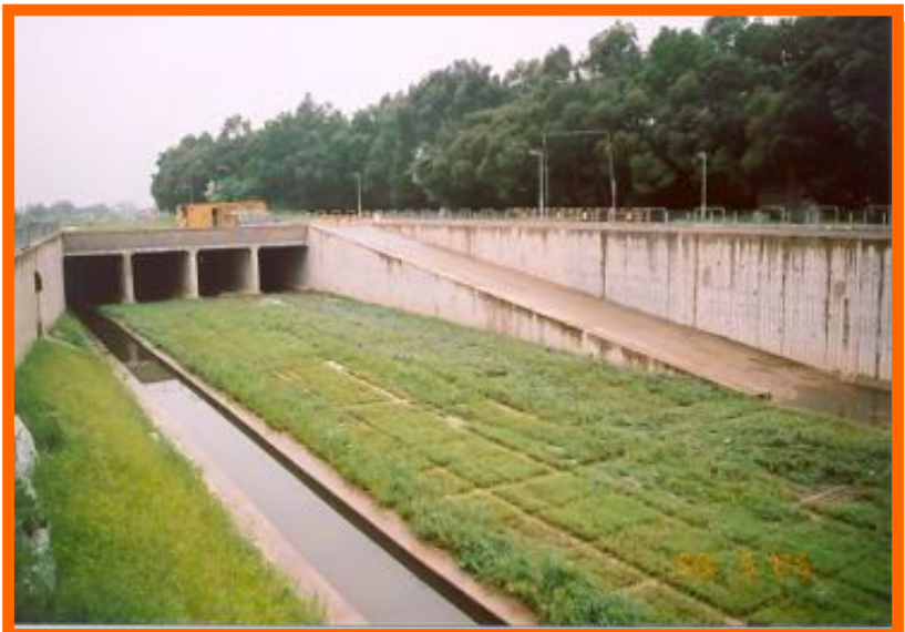
Eco-design: vegetation lines the bottom of the Yuen Long Bypass Floodway.
