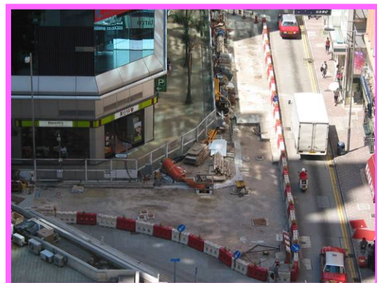
A Meritorious Award was awarded to the contractor who was in charge of Wan Chai East & North Point Sewerage. Site staff set up a proper temporary traffic management system during construction work.
