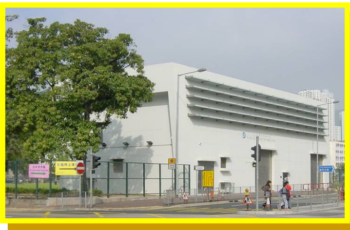
The Tai Hang Tung Floodwater Pumping Station has helped to resolve flooding problems in West Kowloon.
