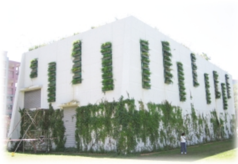
Greening at the Tai Hang Tung pumping station
