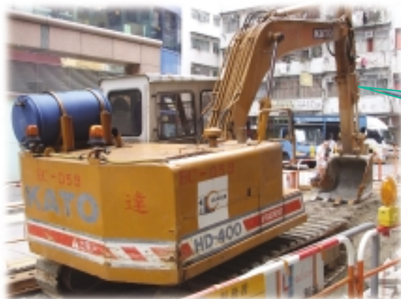
A good example of environmental practice by a contractor - the use of an excavator equipped with water spraying device to suppress dust emission during excavation
