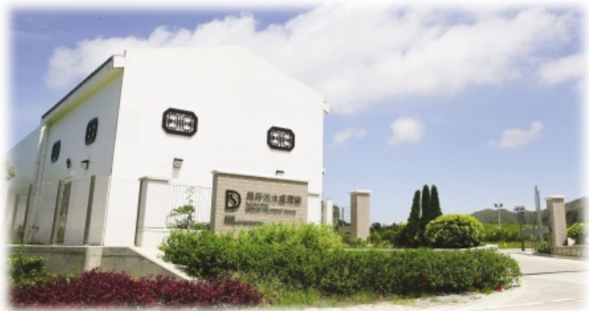
The tertiary sewage treatment plant in Ngong Ping with reclaimed water facilities
