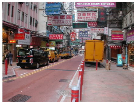
Pilkem Street (footpath widening and streetscape works)
