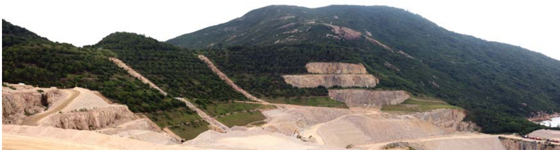
Quarry rehabilitation work in progress
