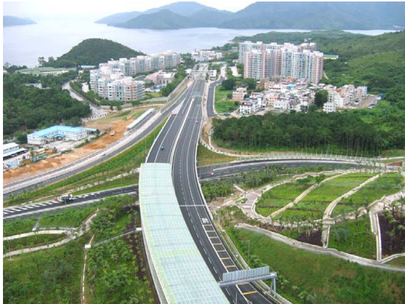
Greening work at Trunk Road T7 – Ma On Shan
