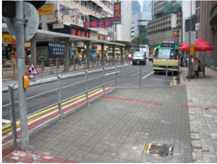
Johnston Road (footpath widening)
