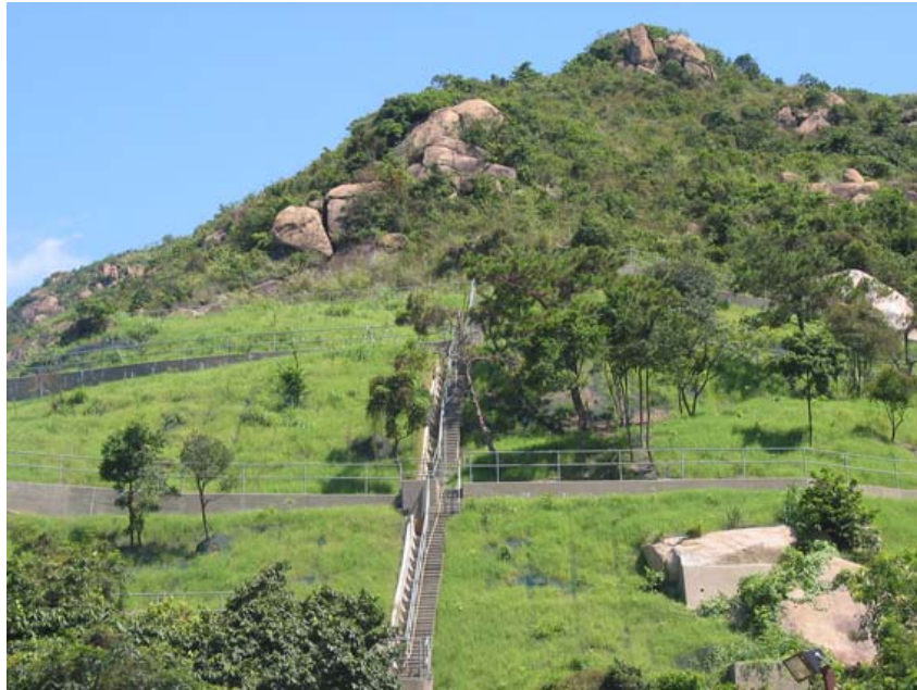
Greening work on one of the LPM slopes – Tsing Yi
