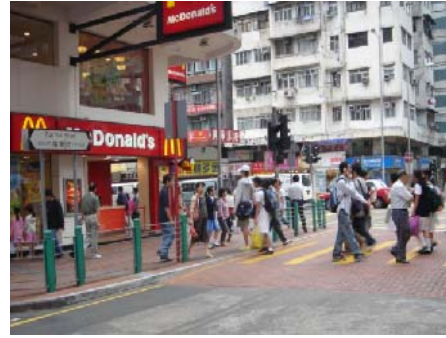
Fuk Wa Street (footpath widening and streetscape works)
