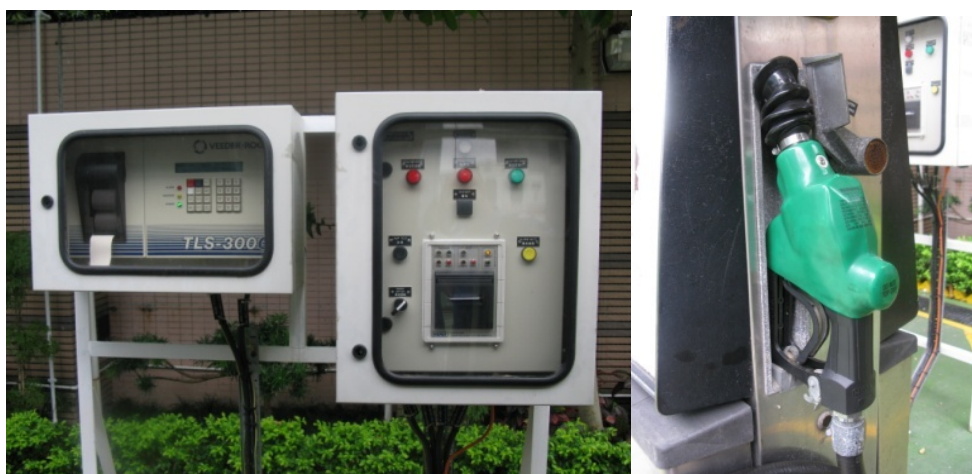
安裝在消防局／救護站的汽油加油站之氣體回收系統 Vapour Recovery System installed at petrol filling station of fire station/ambulance depot
