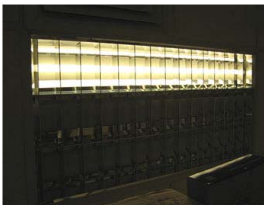
Removal of fluorescent light bulbs in offices and corridors
