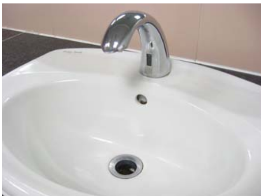
Plumbing appurtenance with water saving devices
