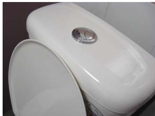
Plumbing appurtenance with water saving devices
