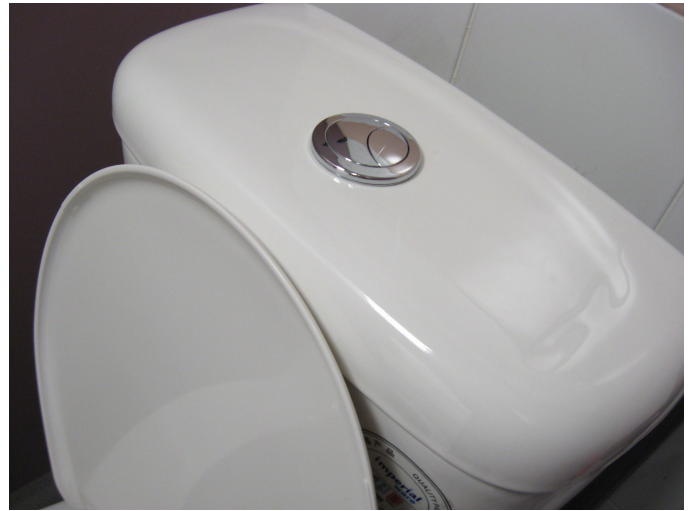
Plumbing appurtenance with water saving devices
