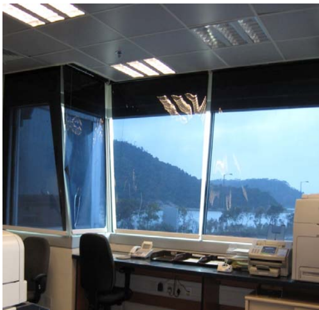
Solar films at the Air Command and Control Centre
