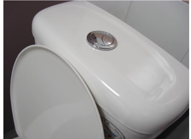
Plumbing appurtenance with water saving devices
