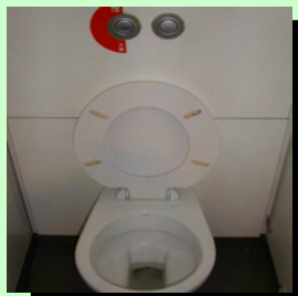
Dual flush / water saving cistern placed in some government offices
