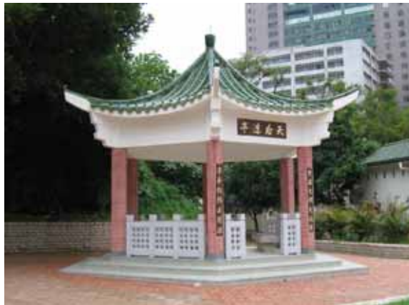
Construction of Pavilion near Tin Hau Road Tuen Mun District
