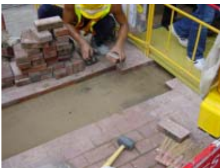
Reinstating the original block pavers after completion of utility work
