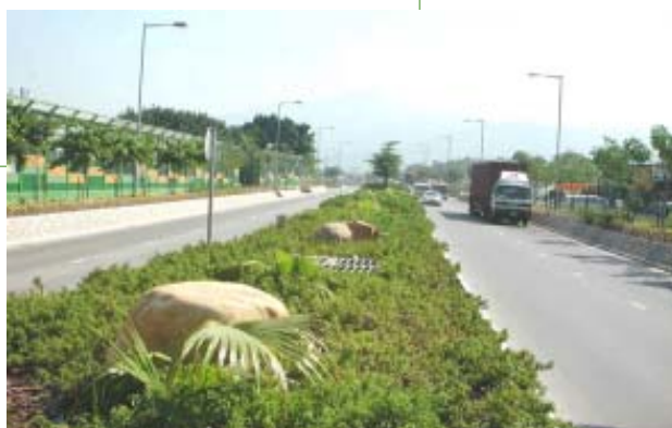
Kam Tin Road widening
