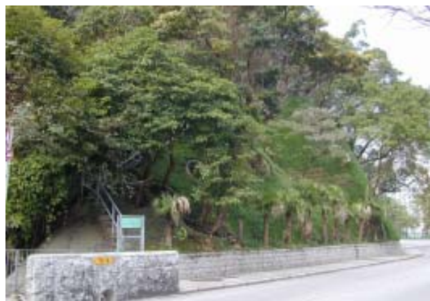
Slope at Tai Hang Road after greening by cellular confinement system
