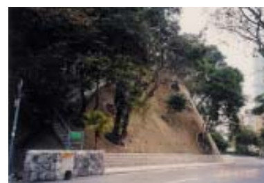
Slope at Tai Hang Road before greening
