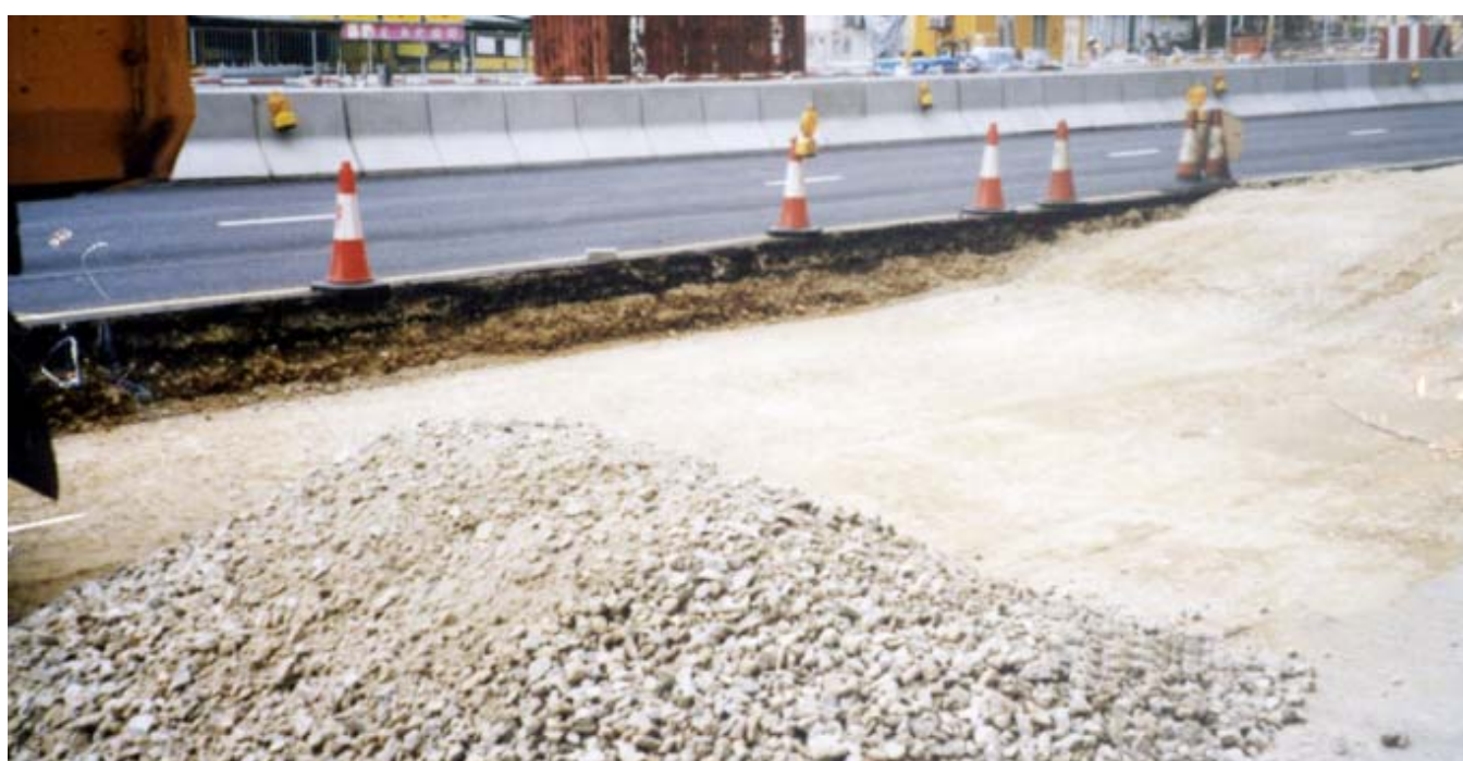
Laying recycled aggregate as road sub-base
