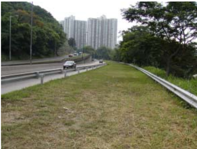
Sha Tin Road (before improvement)
