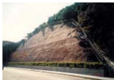
Slope at Wong Nai Chung Gap Road before greening
