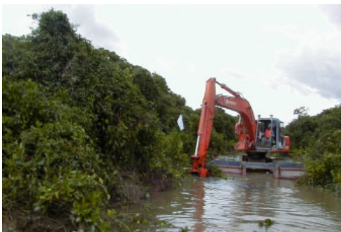
Dredging at Inlet Channel to Gei Wais
