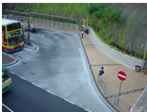
Wah King Street Reconstruction
