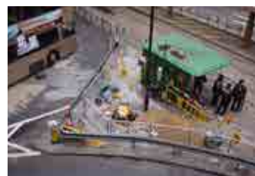
Before near Tram Station (Pennington Street)
