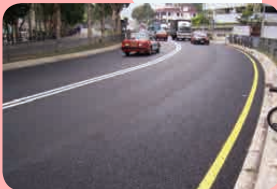
Low noise surfacing at Chui Tin Street, Shatin
