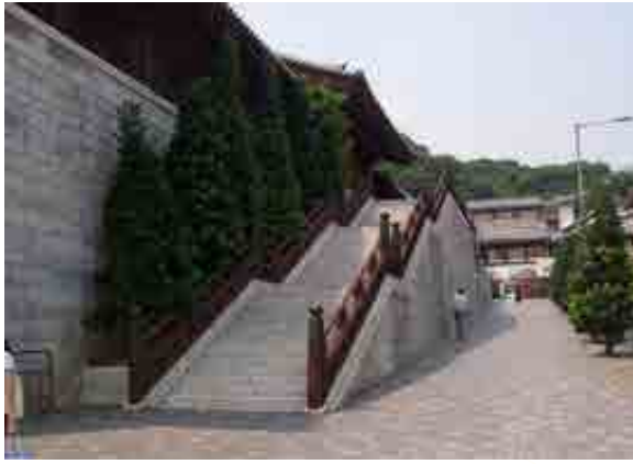
General view at Chi Lin Drive
