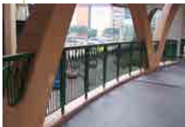
Before Yee Wo Street Footbridge.
