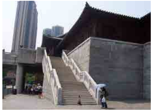
General view at Fung Tak Road
