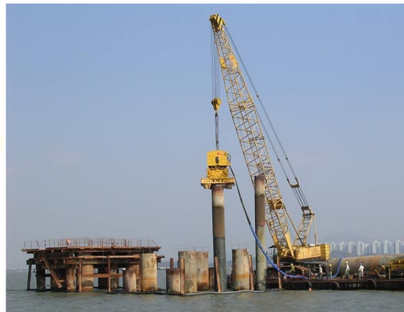
Marine piling using temporary access Bridge
