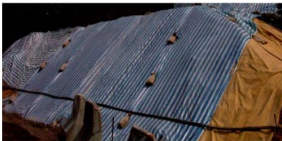
Covering of open stockpiles / temporary slopes
