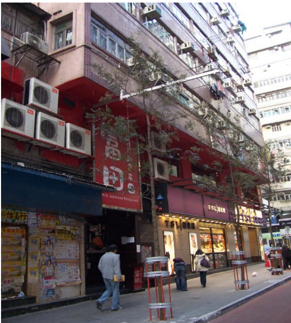
Tree planting of Grevillea robusta , the theme street tree in Nanking Street, Jordan Pedestrian Scheme
