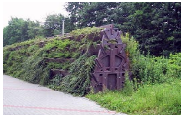
Earth mound using interlocking stacking system
