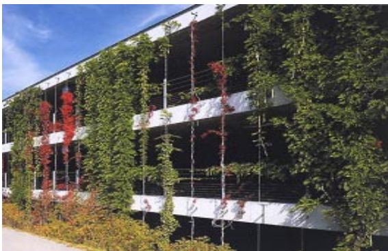
Walls covered with twining climbers on cables
