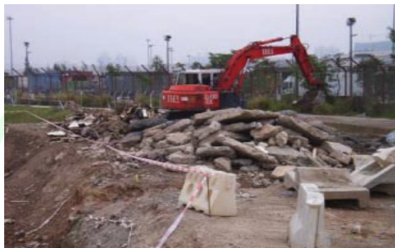
Sorting of non-inert material on site
