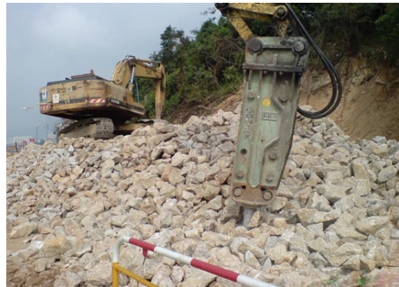
Secondary breaking of rock and concrete to Grade 400 size
