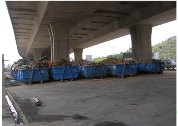
A designated area for the disposal and segregation of construction waste
