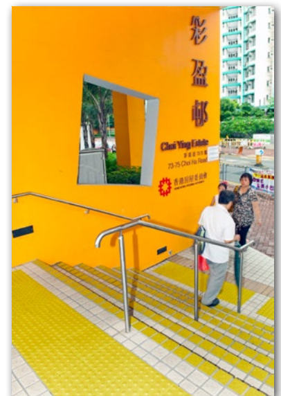
Handrails and tactile warning strips
