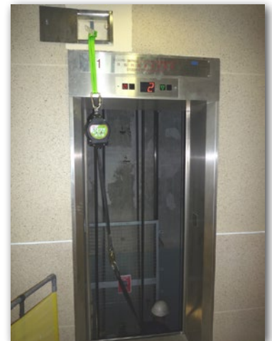
Retractable fall arrestor in use
