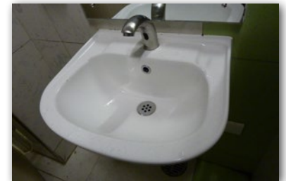
Sensor-controlled water tap
