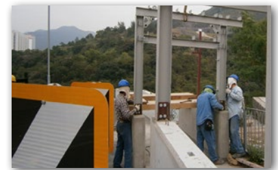
Reusable modular site hoarding
