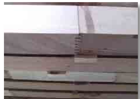
Finger joints in timber doorsets
