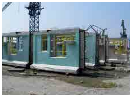
Use of precast concrete component
