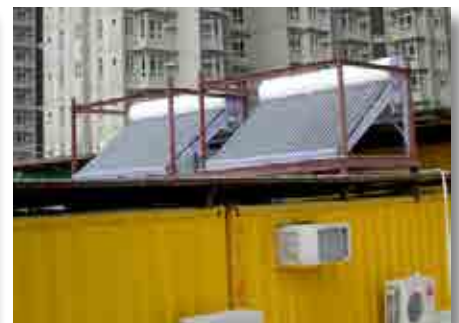
Provision of solar hot water heaters in workers' shower area
