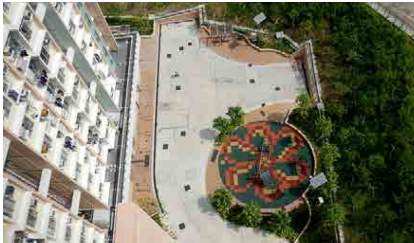
Green treatment for a newly formed slope in Tai Pak Tin Street in Kwai Chung
