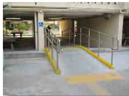
Barrier-free facilities in Oi Man Estate
