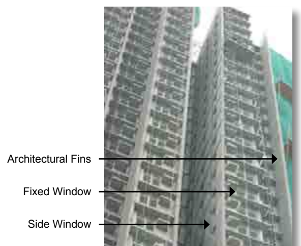
Fixed window facing major noise source and side window for ventilation
