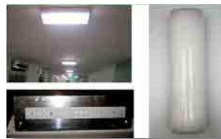
Trial installation of LED bulkheads in Kai Tak Site 1A
