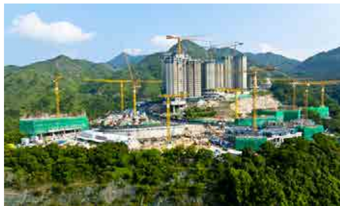
Sha Tin Area 52 Phase 1 project
