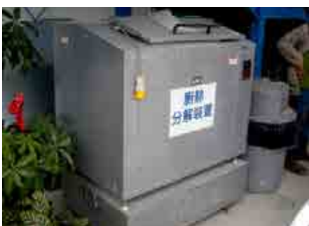
Provision of food waste composting facility at remote locations with site canteen or catering service
