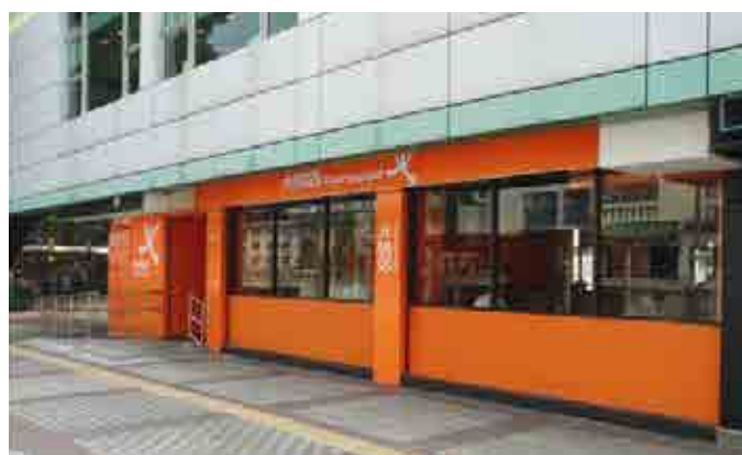
Upgrading works in Wah Fu (I) Estate
