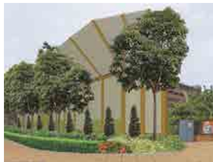
Noise barrier to reduce noise at propagation path
