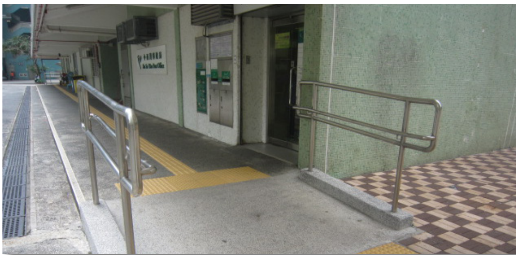
Barrier-free access improvement works in Siu Sai Wan Estate
