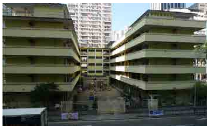
Chai Wan Flatted Factory - Before Conversion
