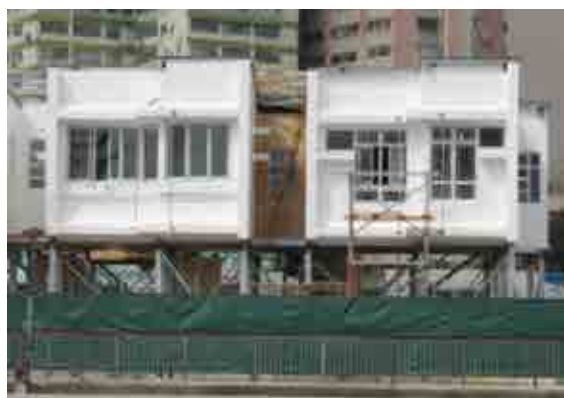
In-situ testing at San Po Kong site
