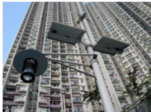
Pole lamps powered by renewable energy
