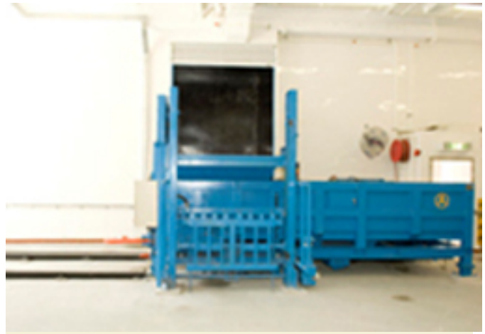
Central Refuse Compactor system
