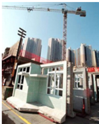
Prefabricated building elements on site
