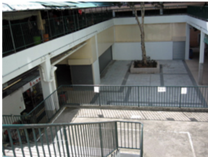
Appearance of Nam Shan Market after Renovation
