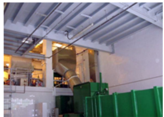
De-odouriser installation
