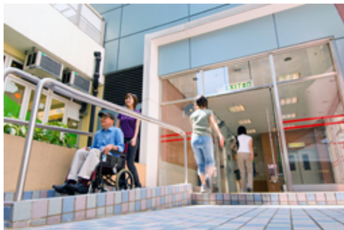
Access ramps and barrier free access
