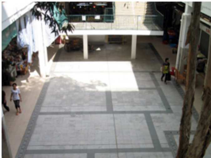
Appearance of Nam Shan Market after Renovation
