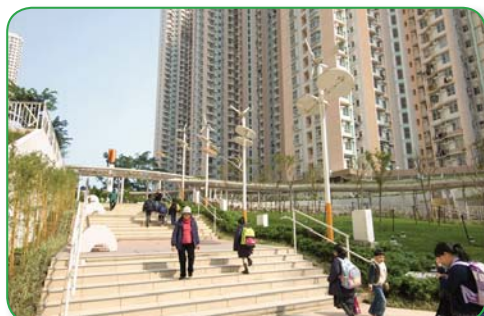
Wind and solar hybrid powered outdoor lighting system in Sau Mau Ping South Estate
