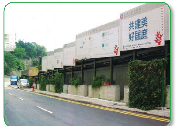
Vertical green hoarding in construction sites
