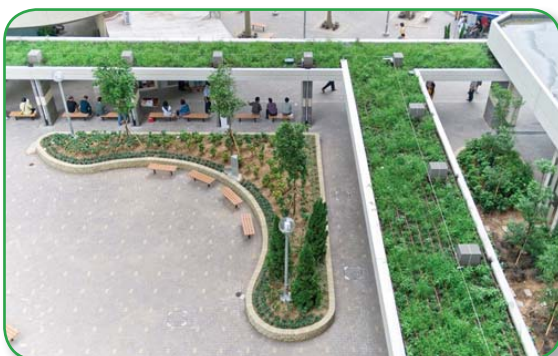
The green roof of the covered walkways in Upper Ngau Kok Estate
