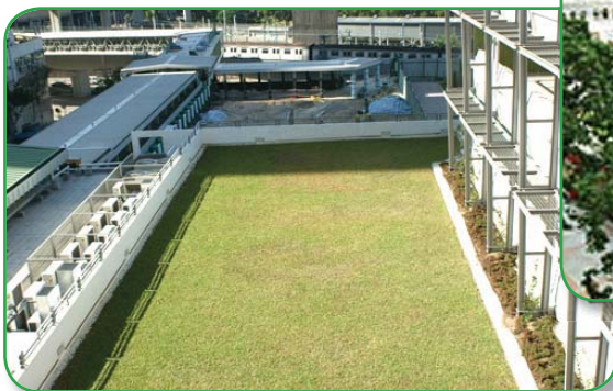
The roof top of the commercial centre in Choi Ying Estate blanketed with turf
