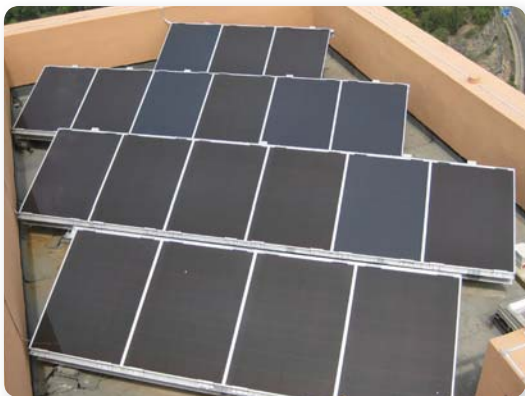
Amorphous Silicon Thin Film PV Modules in Eastern Harbour Crossing Site Phase 5
