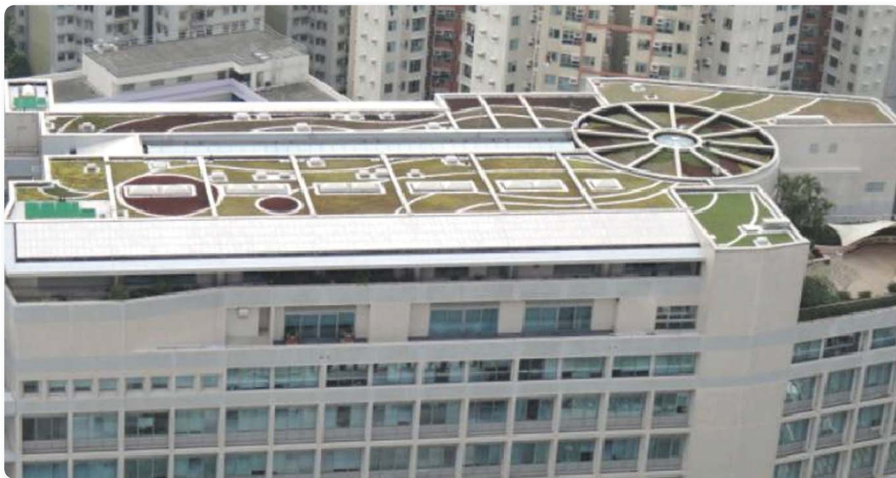
Green Roof at Housing Authority Headquarters
