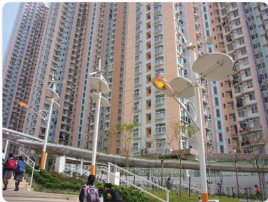
Wind-solar Hybrid Energy Lighting at Sau Mau Ping South Estate
