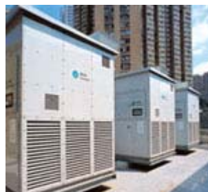
We piloted an energy-saving gas-fired dehumidifying air-conditioning system at Hin Keng Market
