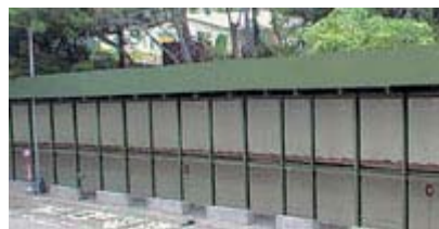
Using re-usable metal hoardings saves timber
