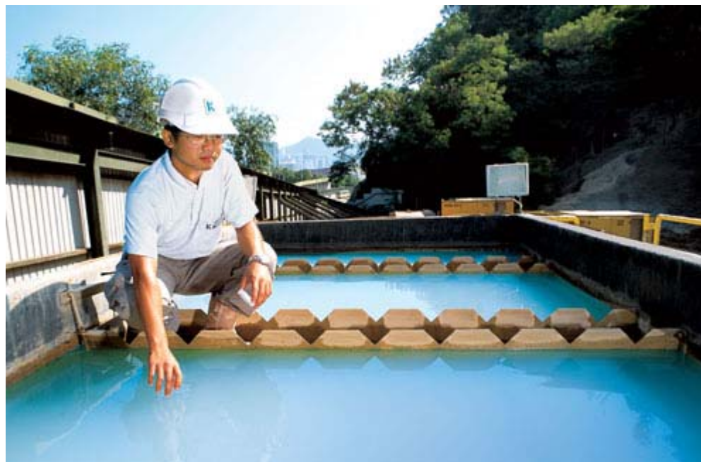
Water Recycling Systems at our piling sites save water
