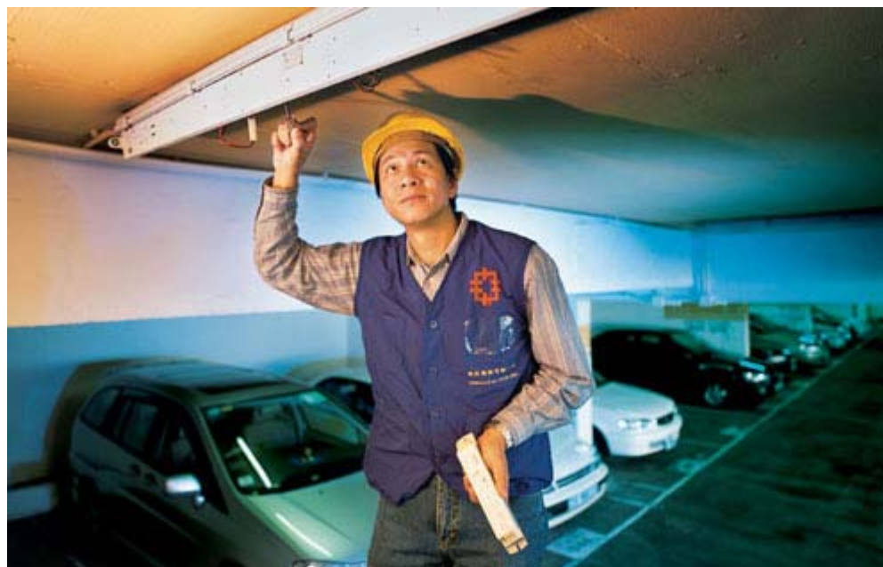
Electronic ballast installation
