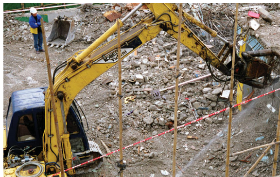
Hydraulic concrete crushers significantly reduce noise nuisance from demolition works
