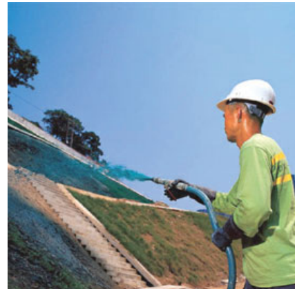
Hydroseeding on estate slope
