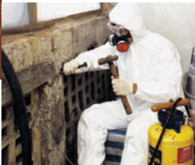
Snapshots of trained workers removing asbestos-containing materials
