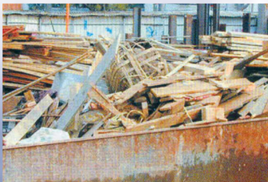
Sorting of construction and demolition waste on site
