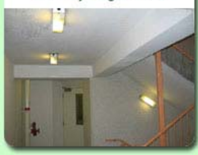
Replacing double lighting tubes by single tubes
