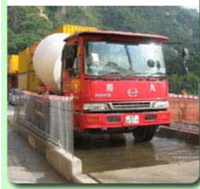
Wheel-washing bay at construction site
