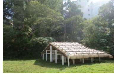
Figure 4: Instrument shed on the lawn of HKO HQ
