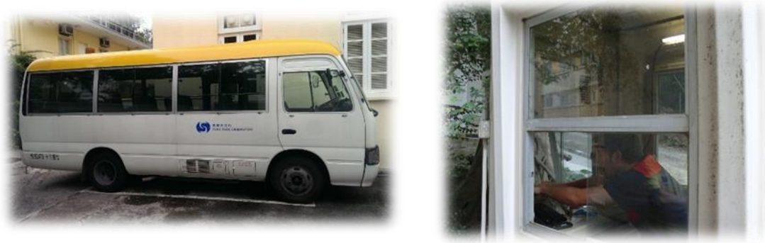
Figure 9: Installing solar film in department vehicle and security guard room
