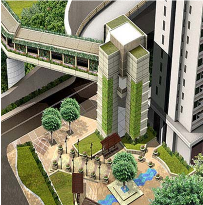
■ Eastern Harbour Crossing Phase 4 Fitted with Vertical Green Panels (under construction)
