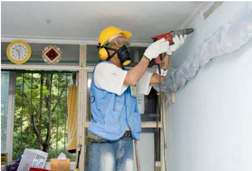
■ Total Maintenance Scheme Repair Activities
