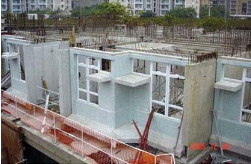
■ Advanced Pre-cast Technology Adopted for Kwai Chung Flatted Factory
