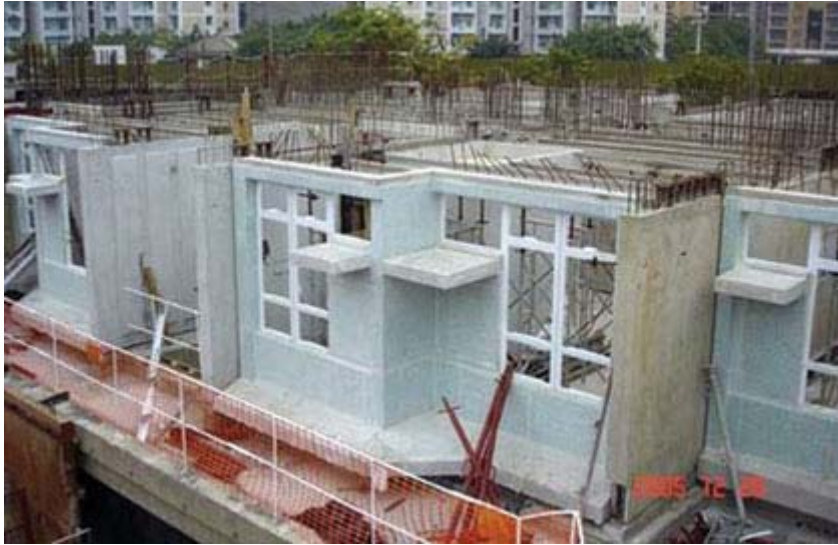
■ Pre-cast Technology Adopted for Kwai Chung Flatted Factory
