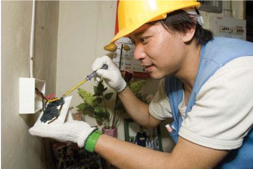
■ Total Maintenance Scheme Repair Activities
