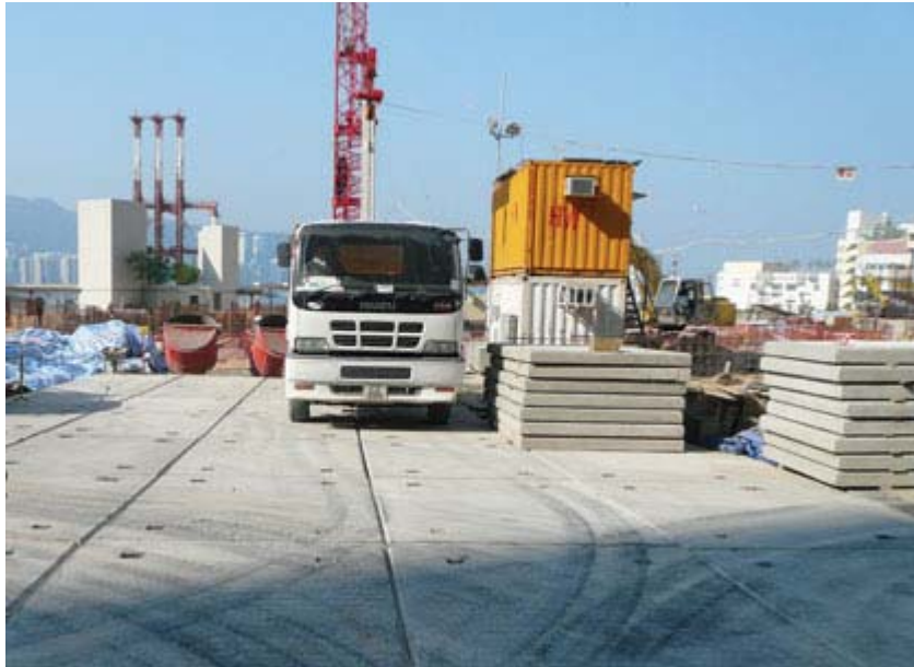
■ Hard Paved Construction at One of Our Construction Sites
