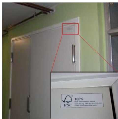
Softwood Timber Doors Installed in PRH Estates
