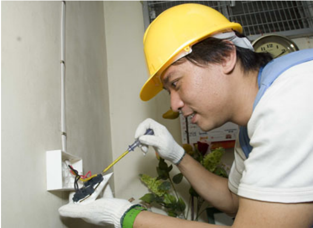
Rewiring inside domestic flats
