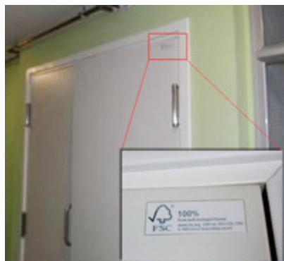
Softwood Timber Doors Installed in PRH Estates
