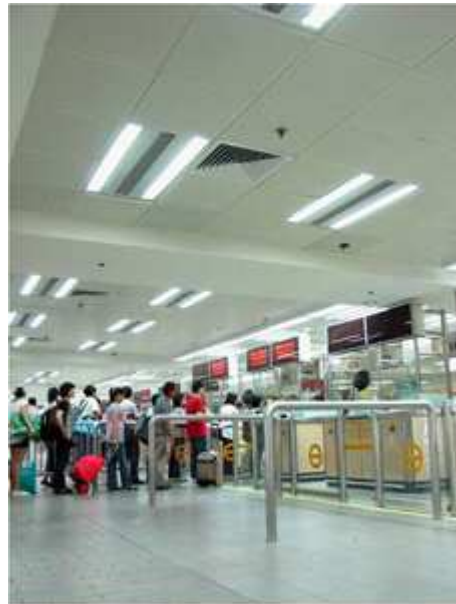
Illumination level of the arrival, departure and visitor clearance halls at Lo Wu Control Point was adjusted to a suitable level.
