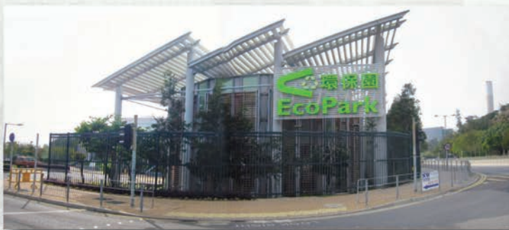
▲ EcoPark in Tuen Mun Area 38
