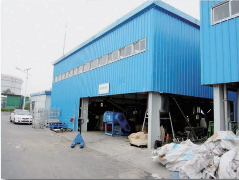
▲ Plastic Resources Recycling Centre at EcoPark
