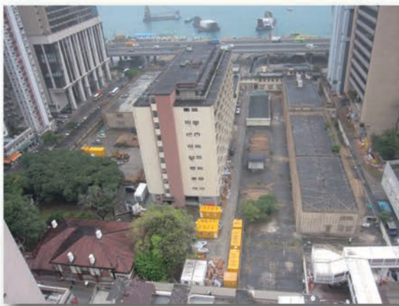
◀ A site with new measures to foster a quality and sustainable built environment at Oil Street, North Point
