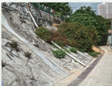
◀ Before slope improvement work
