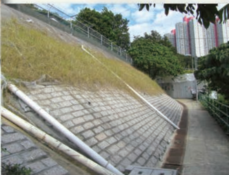
After slope improvement work
