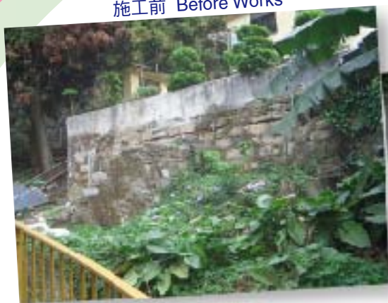
施工前 Before Works
