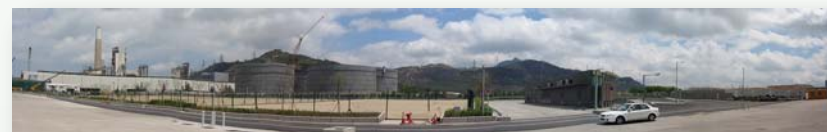
EcoPark in Tuen Mun Area 38
