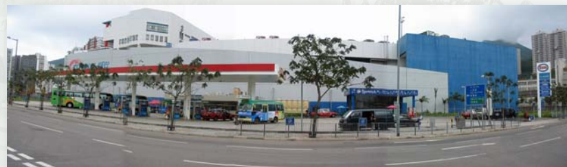
A Petrol Filling Station with LPG filling facilities at Sheung Mau Street, Chai Wan
